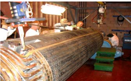
Rotor Rewinding at GMS Facility
