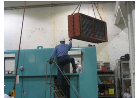
Installation of Refurbished Cooler
